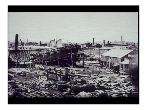
And indeed you try to find out where is the shipyard and what did that look like? In this case in the very early pictures of a shipyard in Baltimore tells a lot of the story. That you see two U-shaped bottom vessels. These are cargo vessels being built. You see the steam box for bending the planks that they go around the hull. And the next step is translate some of that to the vessel you are working on. The look at that steam box, look at the boats.
