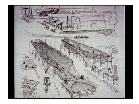
There we've got the steam box again. And we don't have a U-shaped bottom, we've got V-shaped bottoms of the two vessels built for the opium trade. One was the Frolic and the other sister vessel the Dart. It is important to try to reconstruct things as best you can. If you're going to get the information back to a public.
